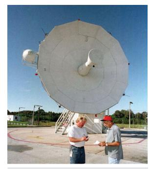
Above, the 9-meter antenna communicates with the shuttle orbiter during launch, in low-Earth orbit and during landing.
